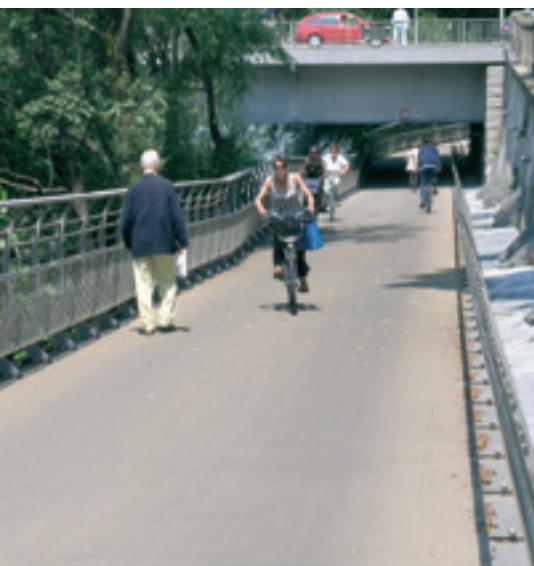
The E. Steininger-Steg is the longest bridge in Graz.
